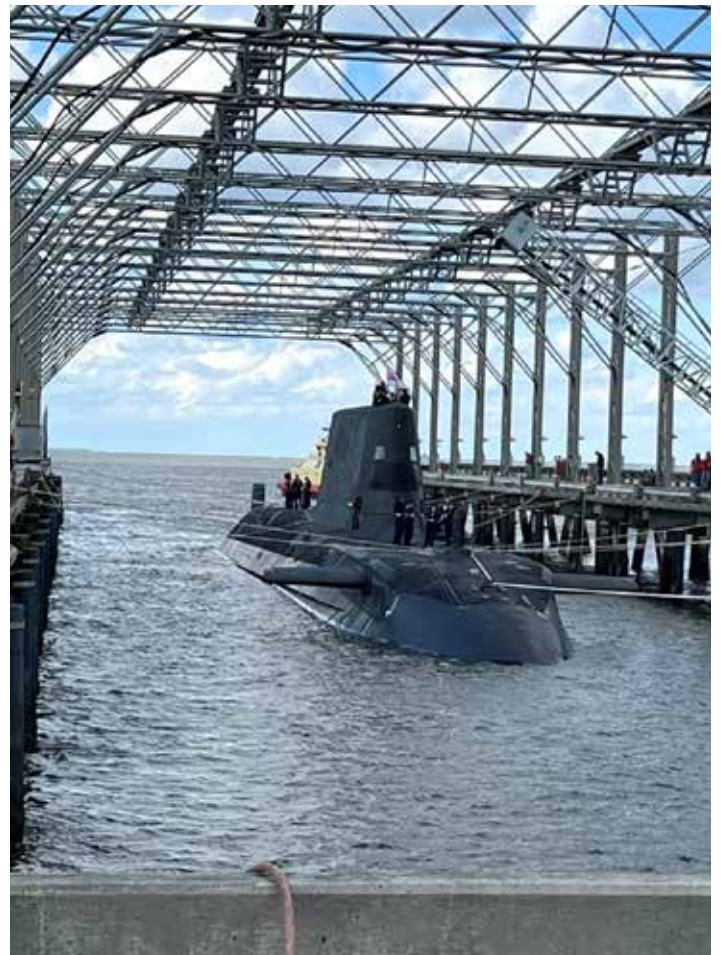
HMS ANSON in the Magnetic Silencing Facility (MSF).
